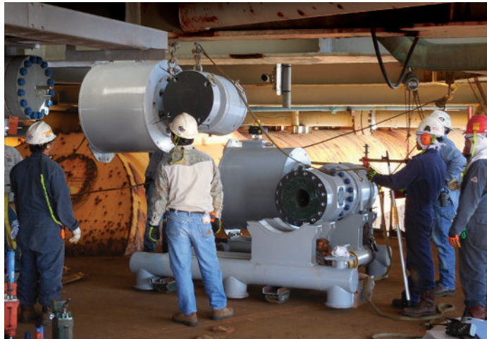
10" x 7-1/16" API 10K complete BSDV Boarding Shutdown Valve skid
